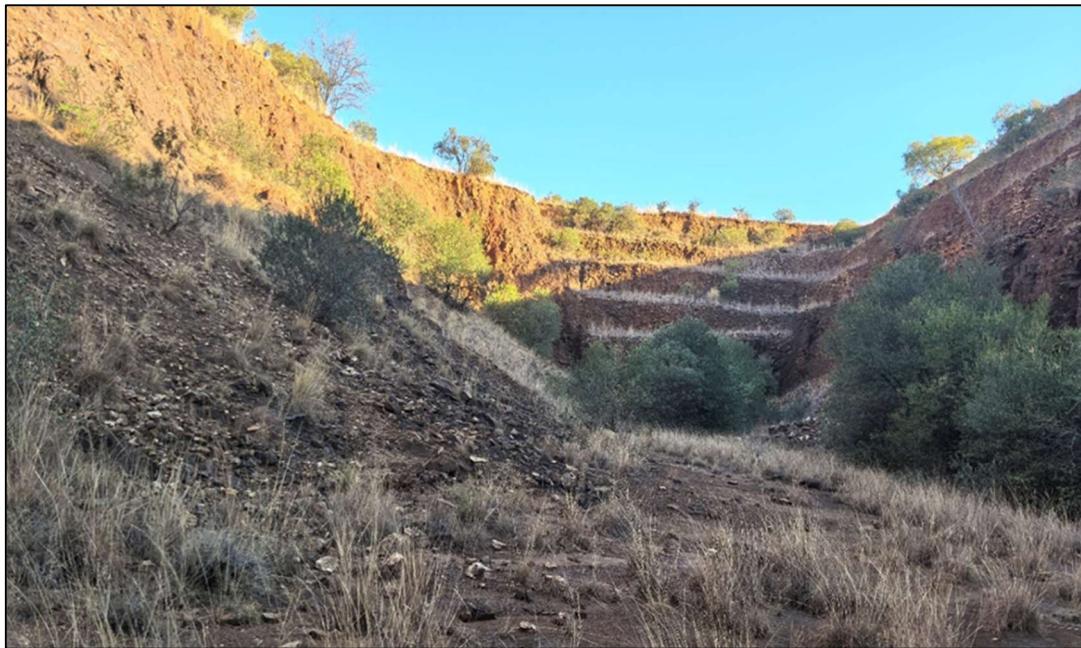
Figure 3: Main pit, southern end
